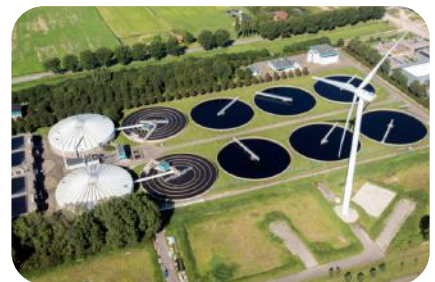
Industrial Water Treatment
